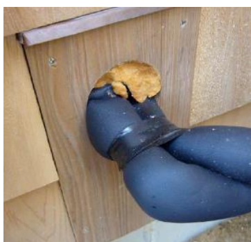
Envelope penetration not sealed properly
