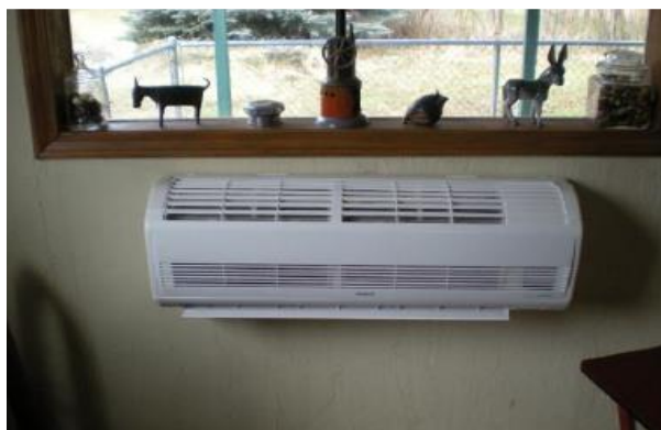
Exhibit 22: Bad Location for Ductless Indoor Unit
