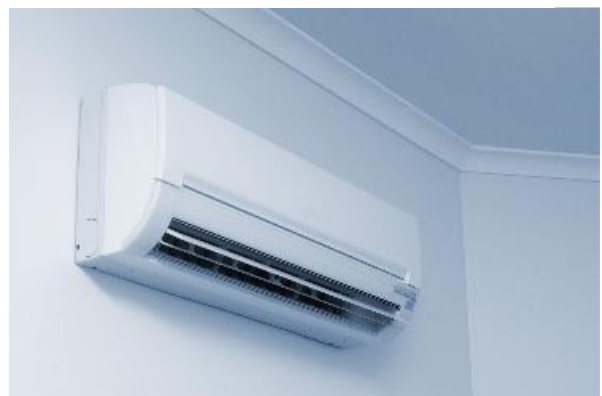
Exhibit 27: Properly Installed Ductless Indoor Unit
