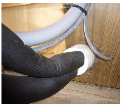
Envelope penetration properly sealed
