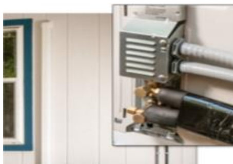
Line set properly insulated
